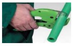
1.) Cut the pipe perpendicular to its axis
